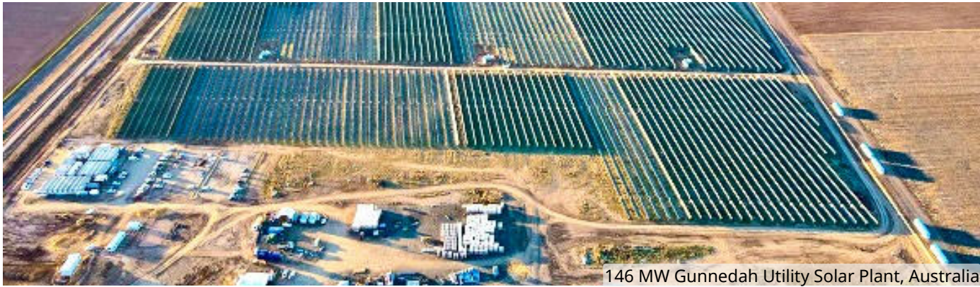
146 MW Gunnedah Utility Solar Plant, Australia
